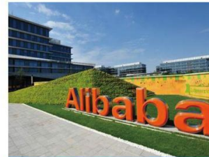
Alibaba Deqing computer room project
