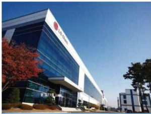
LG Nanjing automobile battery factory
