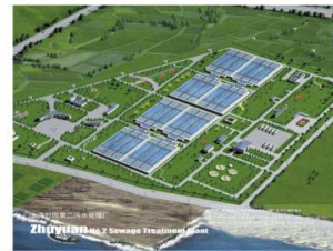
Shanghai Zhuyuan sewage treatment plant
