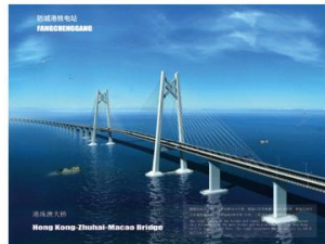
Hong Kong-Zhuhai-Macao Bridge
