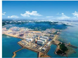
Fangchenggang nuclear power station
