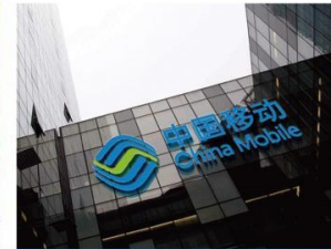
China Mobile Shanghai Jiading project
